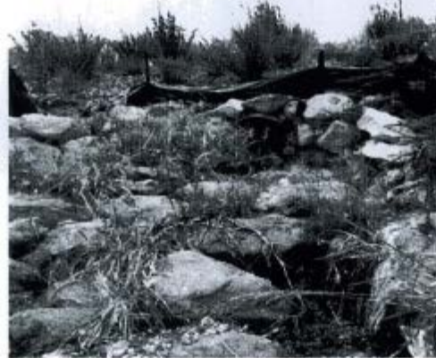
Figure 2: Rip-rap outlet structure with vegetation growing in voids between rocks.
